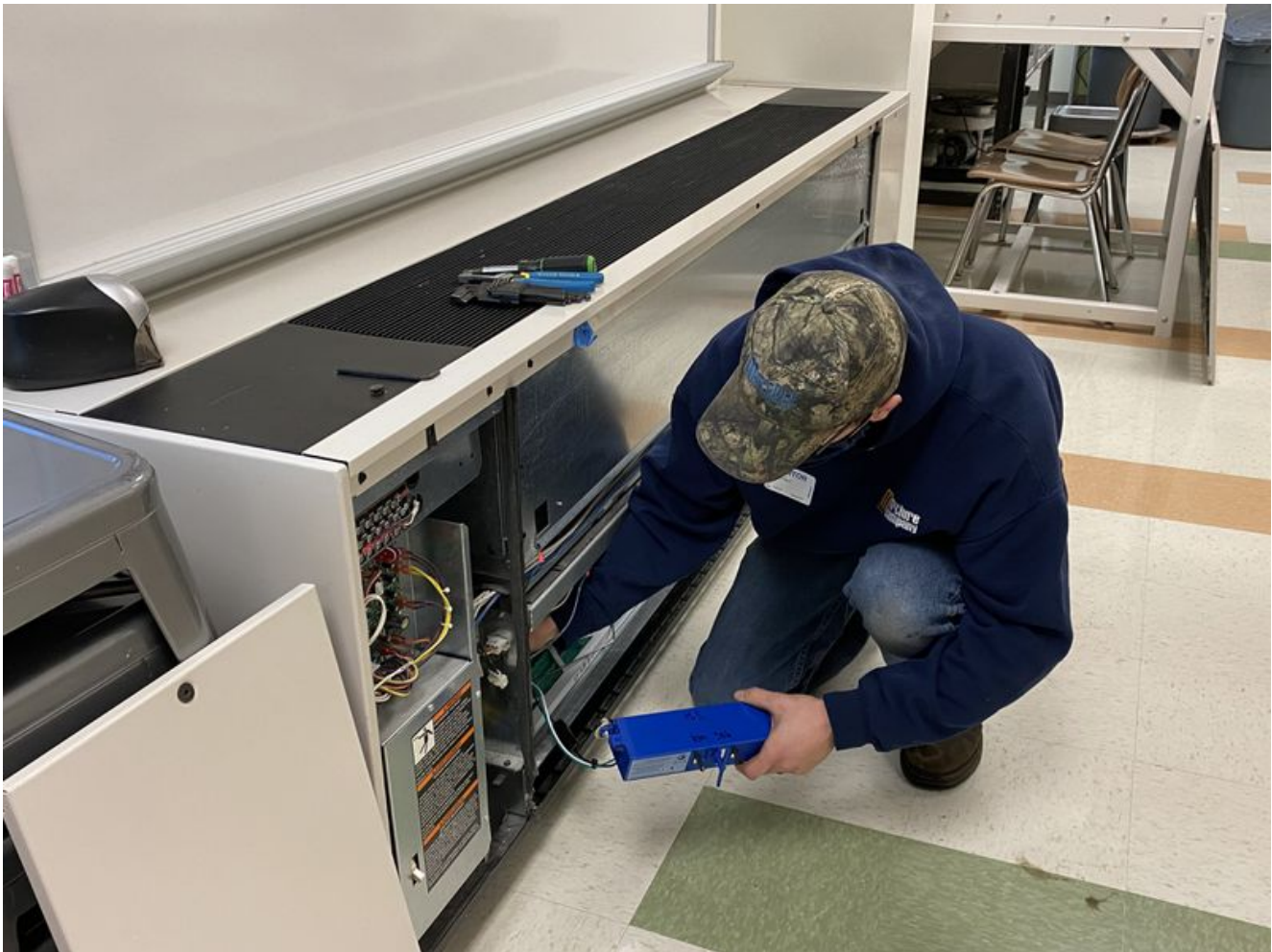
Tim Kopiak of McClure Co. installs a bipolar ionization unit in the HVAC system in a classroom of Northwestern Lehigh High School in early January. (Contributed Photo/Northwestern Lehigh)
